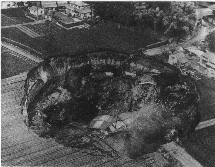
Fig. 12. Collapse of the covering earth layer over the cave made by curring the Oya-stone in Tochigi Prefecture. Excitingly typical solution of iso-perimetric problem in variation calculus. The photo by Asahi Shimbun Publishing Company just after the occurrence on February 10, 1989.
