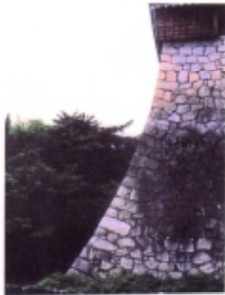
Photo 2 "Sori" curve of the jacket wall
